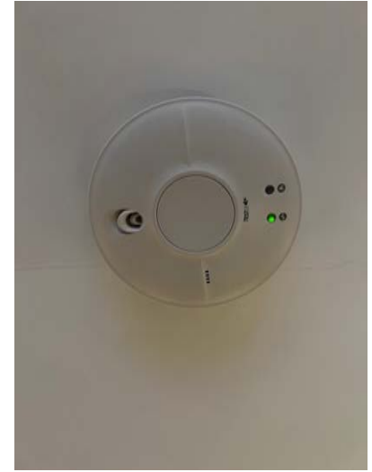
Wired smoke detection
